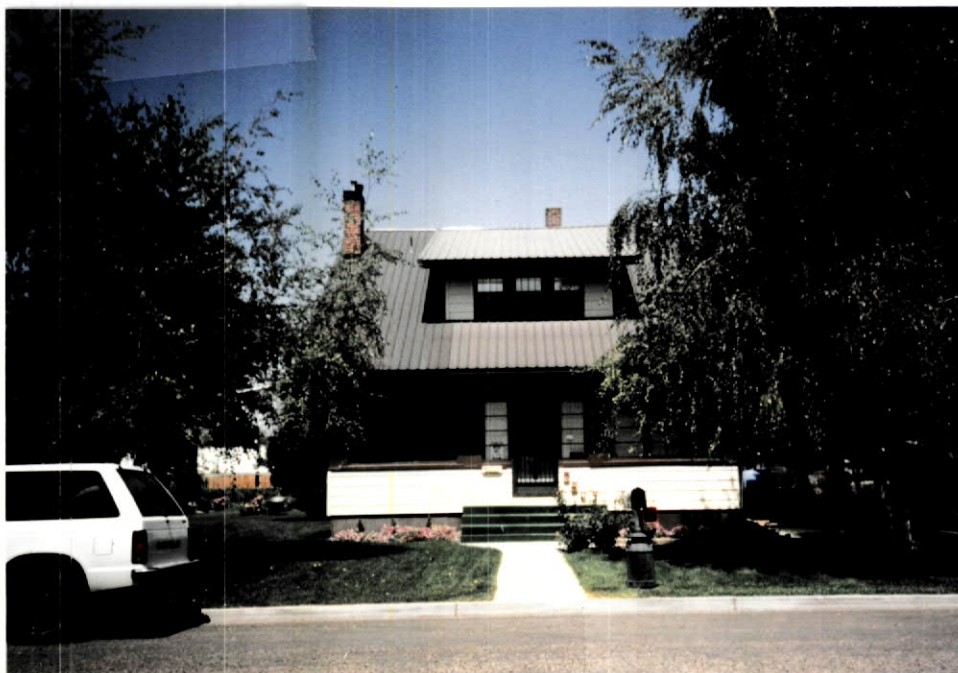
VIEW TO THE NORTH.
