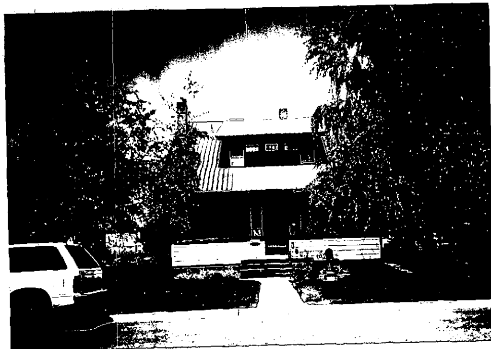
VIEW TO THE NORTH.
