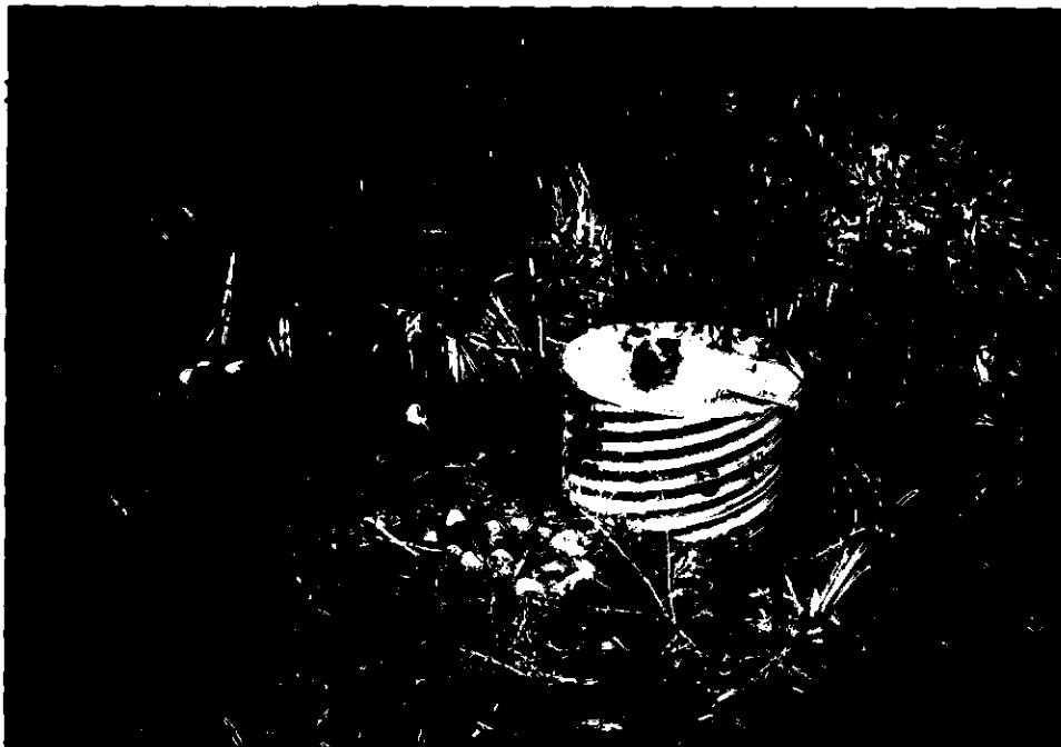
VIEW OF COLLECTION BOX #2. THE WATER SEEPS FROM A SMALL COLLECTION OF SPRINGS LOCATED AROUND THE BOX INTO A 3/4" LINE THAT, THROUGH GRAVITY, FEEDS A STOCK TANK.
