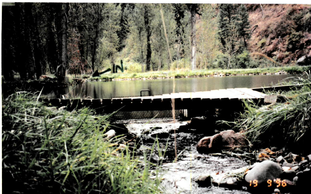
Pond outlet Meas. taken in cement Structure w/ Screen removed. Inlet on opposite side
