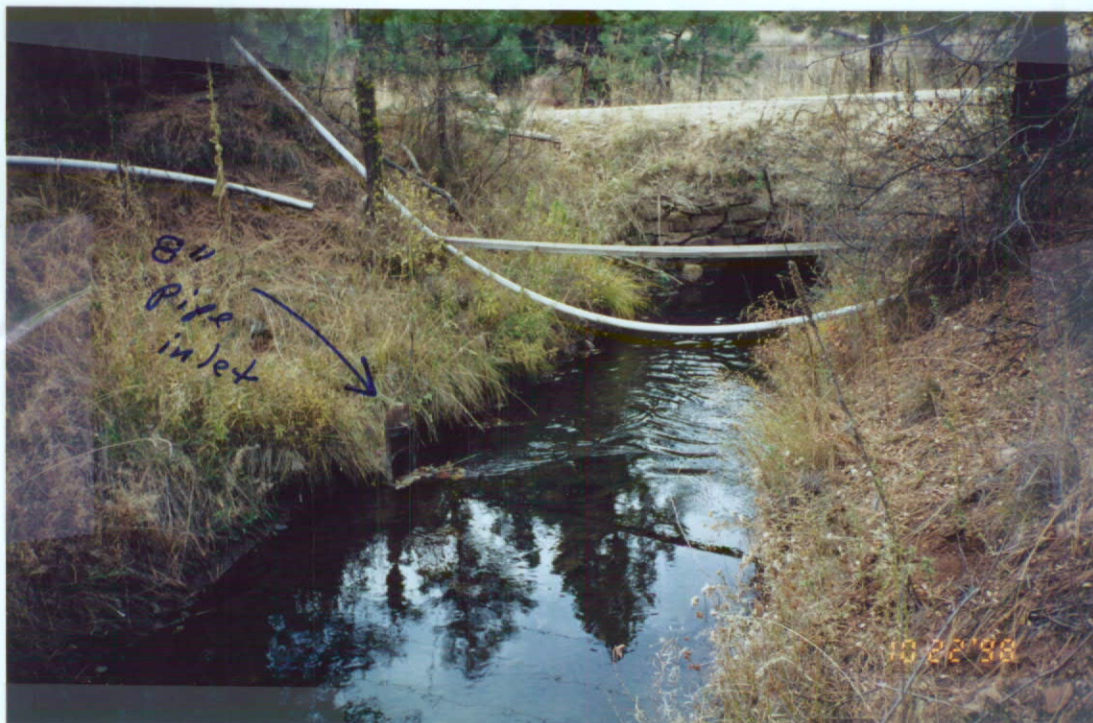
Bear Cr. Rd. Culvert in Background.
