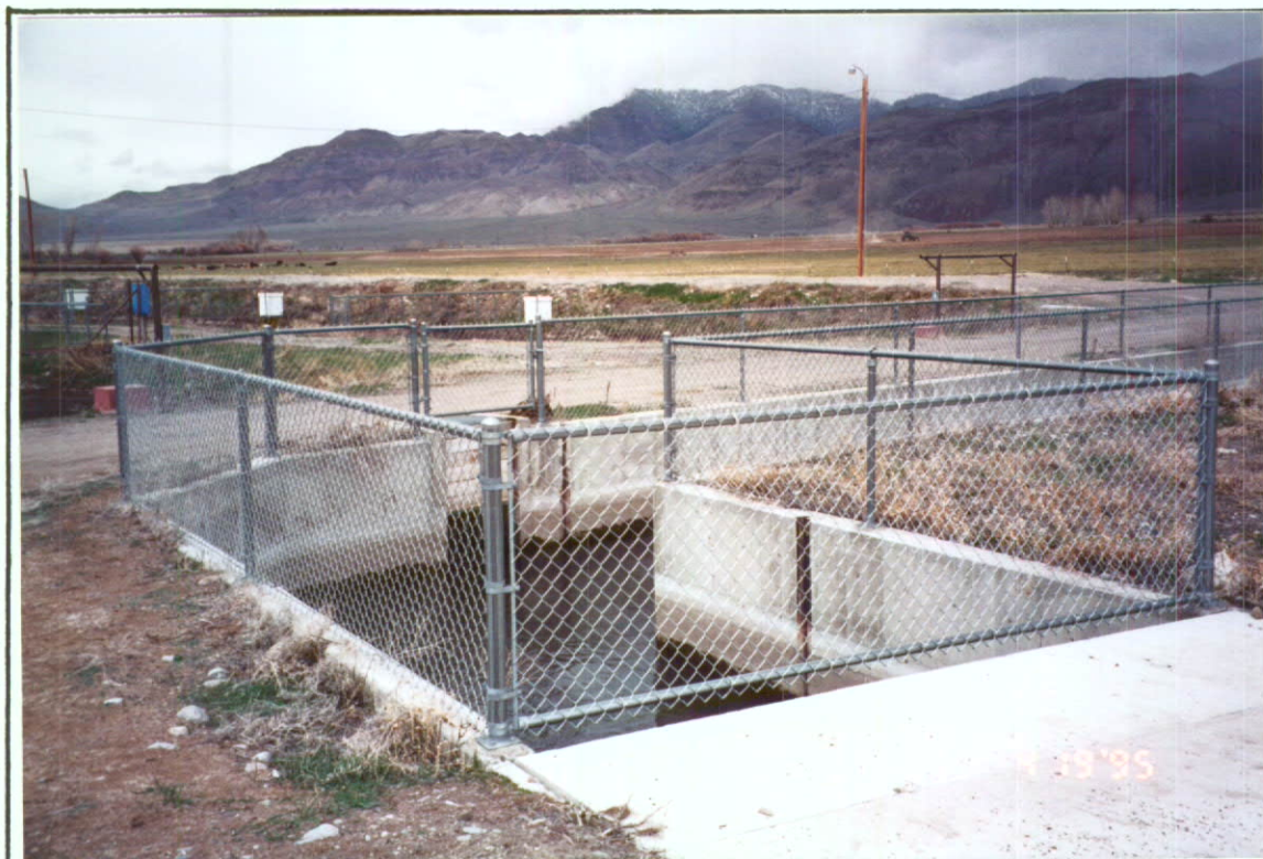
CONCRETE DIVERSION CHANNEL AND GATES TO REARING PONDS.
