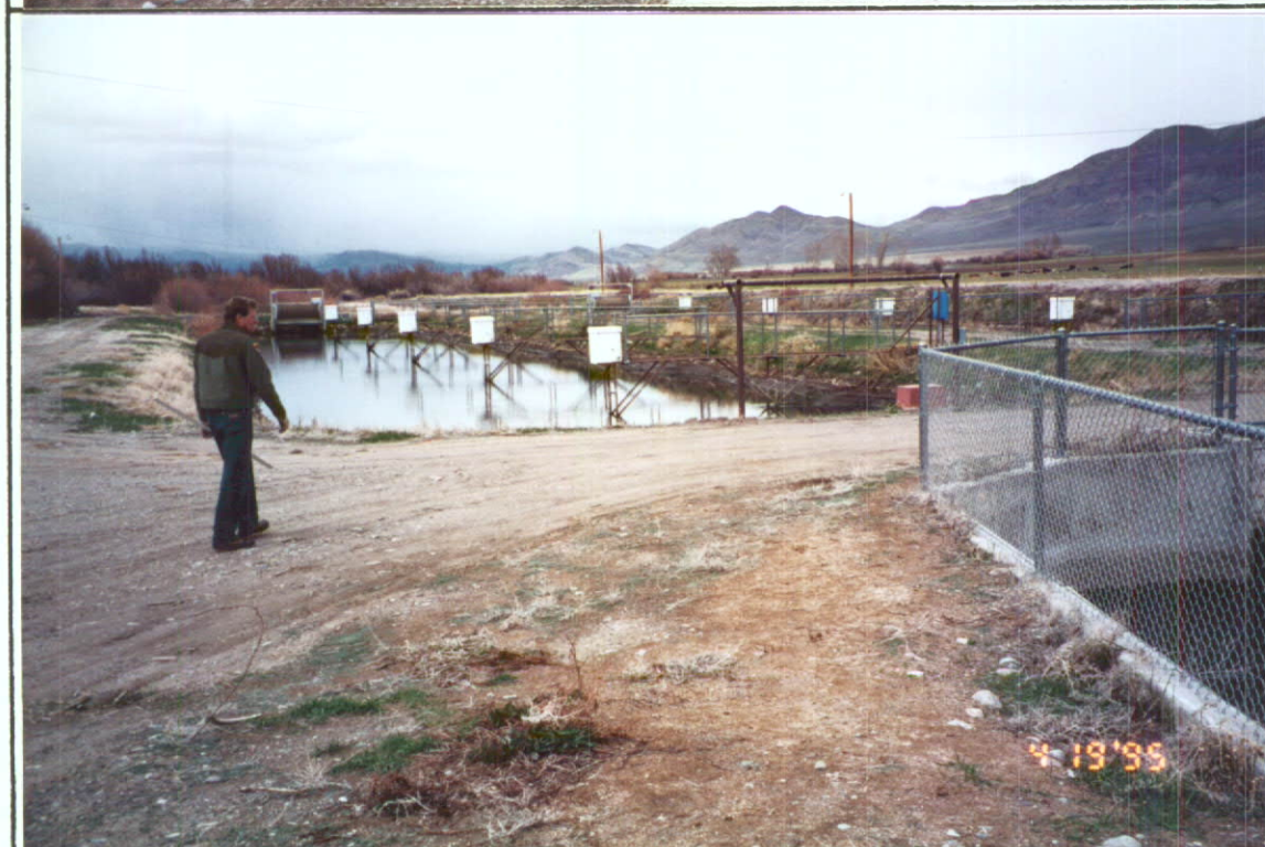
FIRST SET OF REARING PONDS, NORTH OF CONCRETE CHANNEL.
