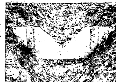
Looking downstream on installed 90° V notch weir. Note end and bottom contractions and weir scales painted on weir plate
