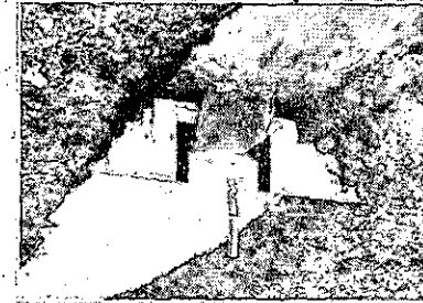
Looking upstream on installed weir. Note the gravel and rock protecting apron and the staff gauge location and staff gauge location
