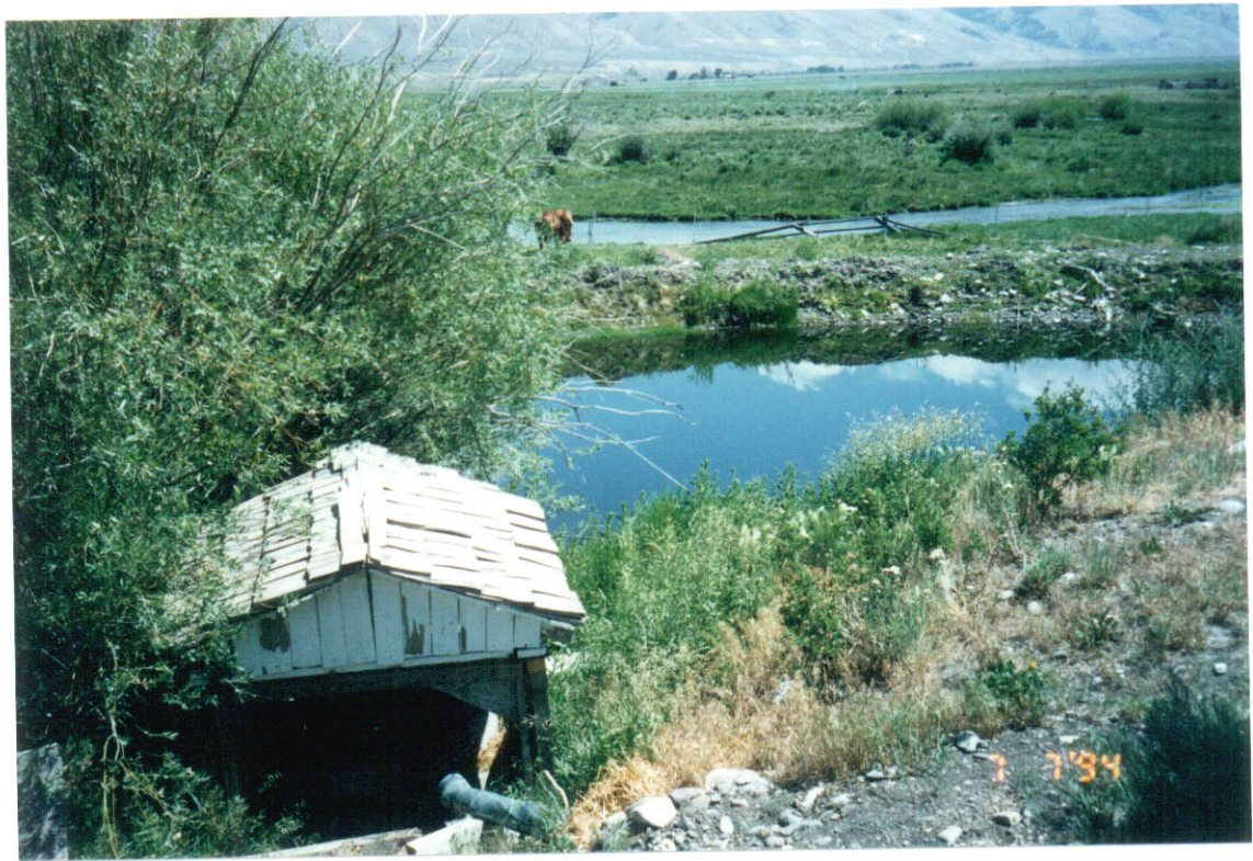
WELL HOUSE (PUMP HOUSE) - EAST OF RESIDENCE LOOKING EAST
