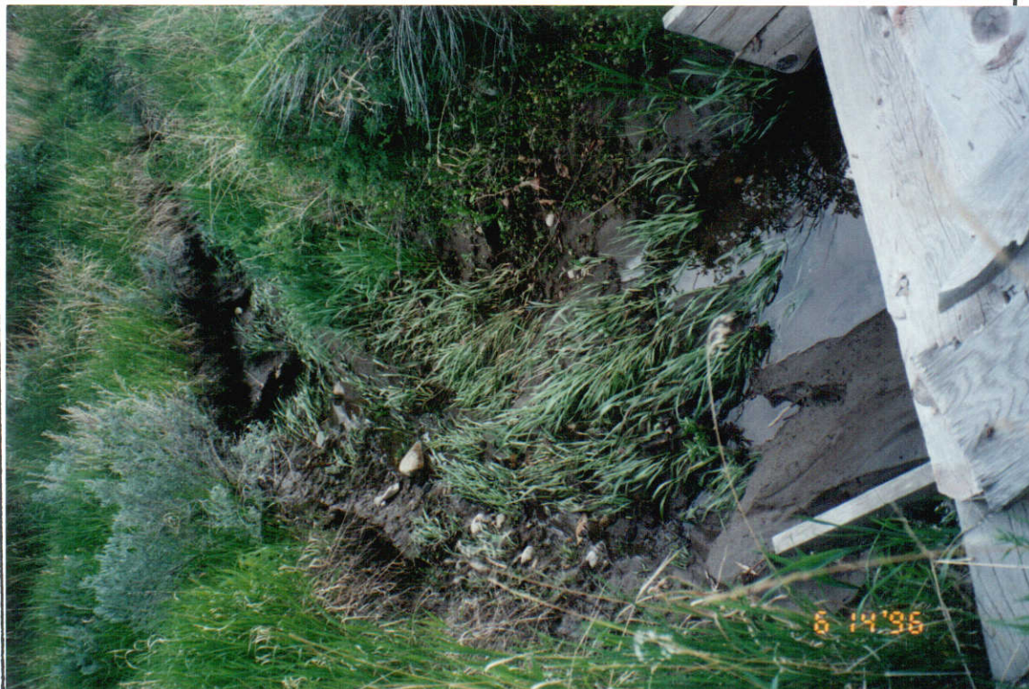
VIEW OF DITCH AND INDICATIONS OF WATER FLOW + USAGE
