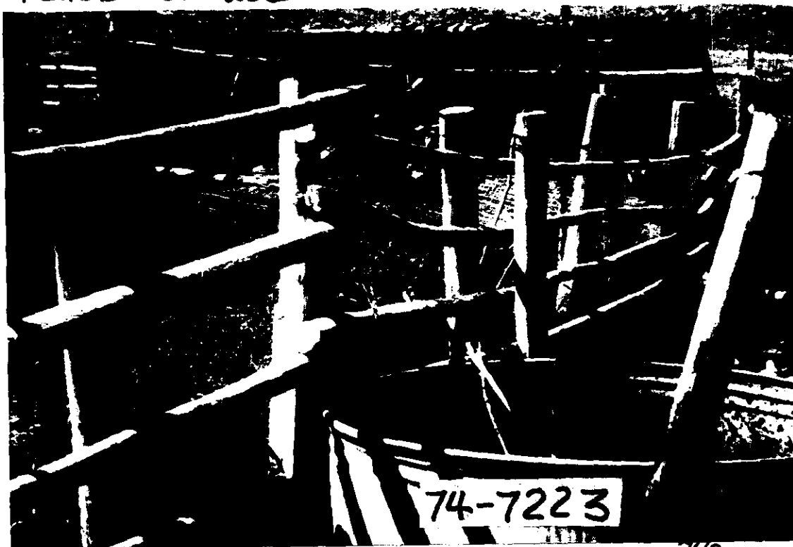
VIEW NORTH AT EAST SIDE OF HOUSE PLACE OF USE
