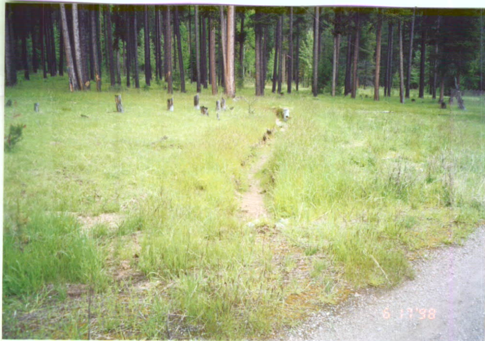
Ditch leaving splitter in culvert to upper portion of Hansen property
