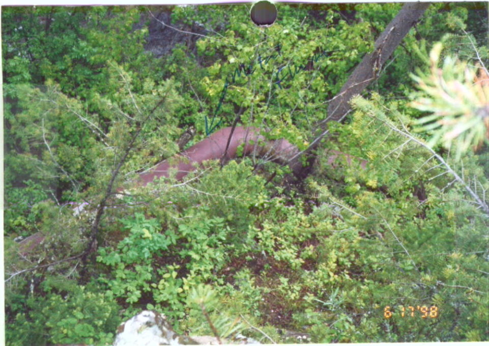
Metal pipe from abandoned N. Fork Diversion
