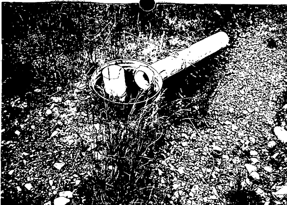
Splitter in Culvert for power + irrigation water from State Creek
