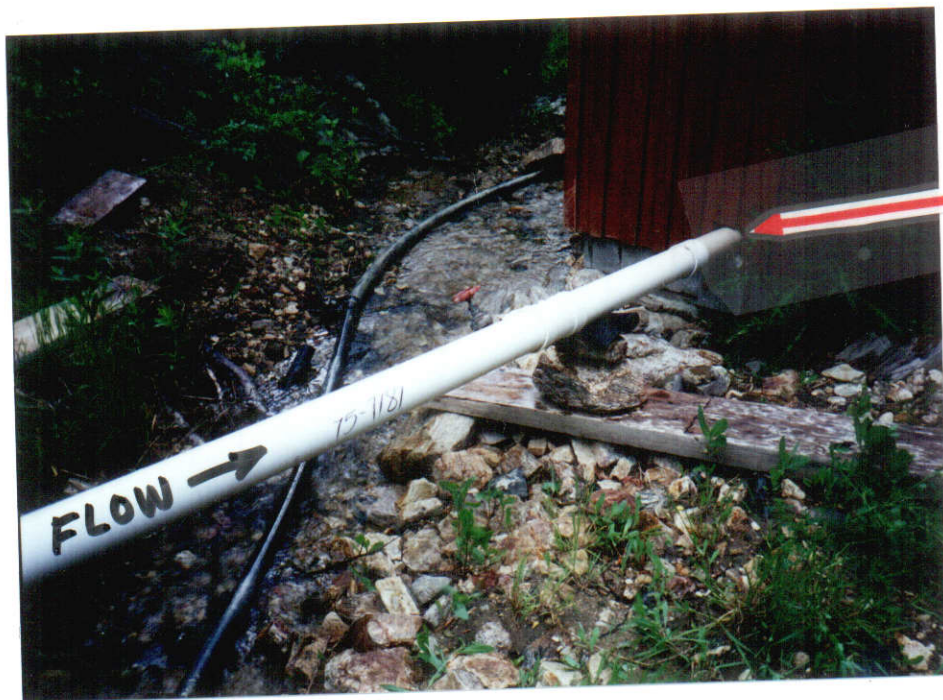
INLET TO POWER HOUSE
