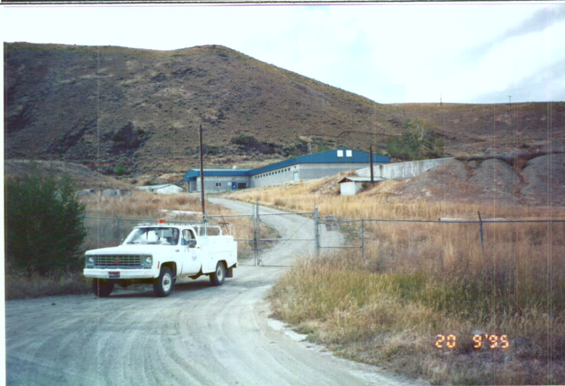
WATER TREATMENT PLANT ABOVE CITY OF SALMON
