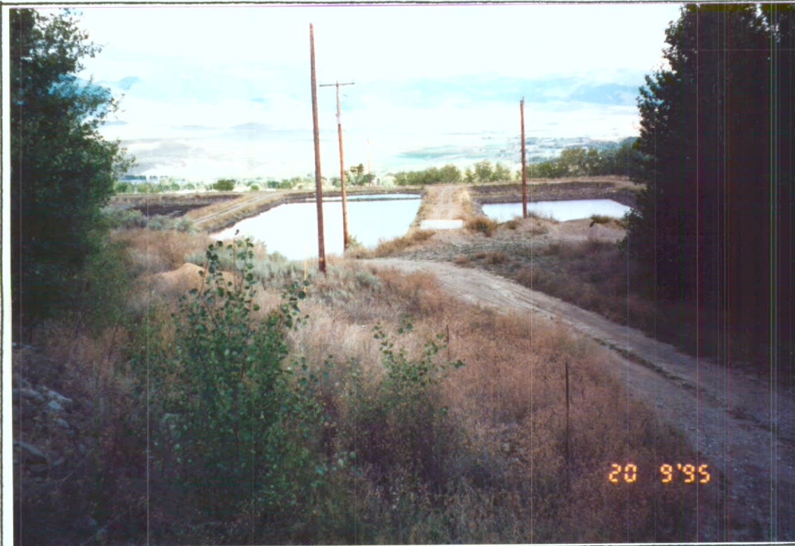
WATER STORAGE PONDS ABOVE WATER TREATMENT PLANT
