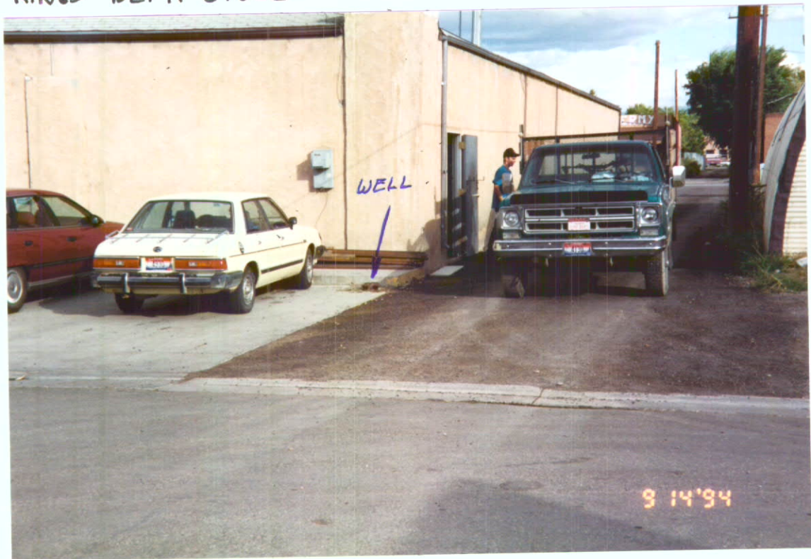
VIEW OF WELL NORTH WEST CORNER OF BUILDING. KINGS DEPT. STORE
