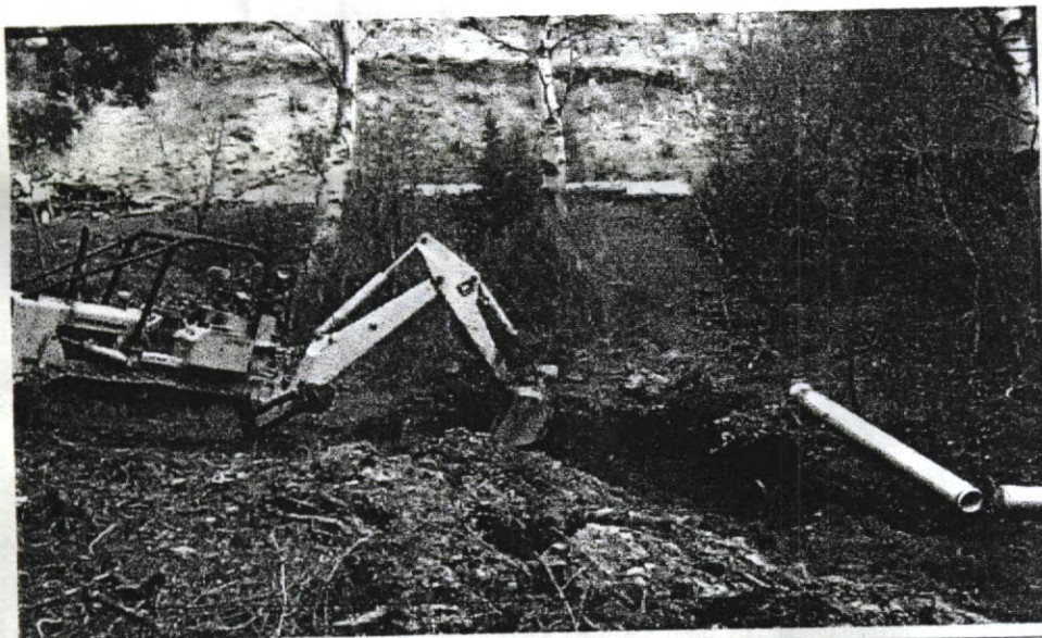
PHOTO # 3 EXCAVATION OF PART OF LAKE CREEK SPRING BY BILL SALO WITH BACKHOE IN SPRING OF 1998
