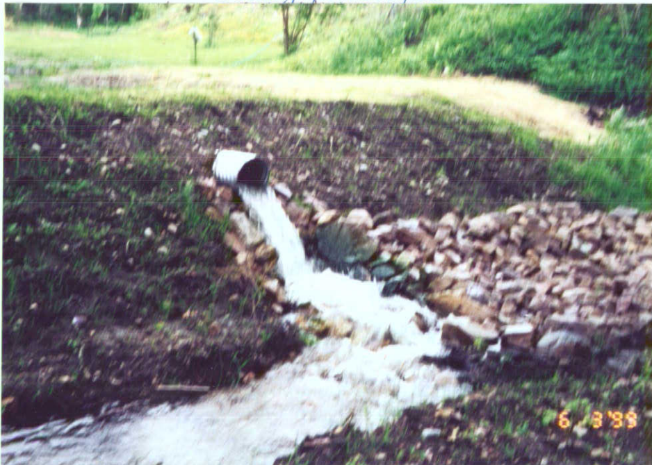
Discharge from Overflow
