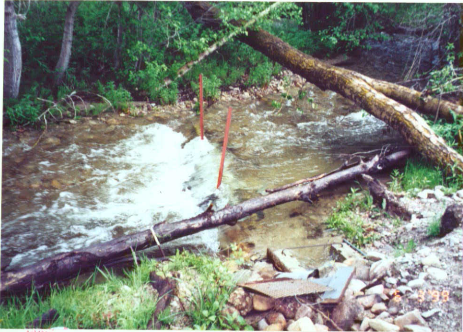
Diversion Dam & Inlet to Pond
