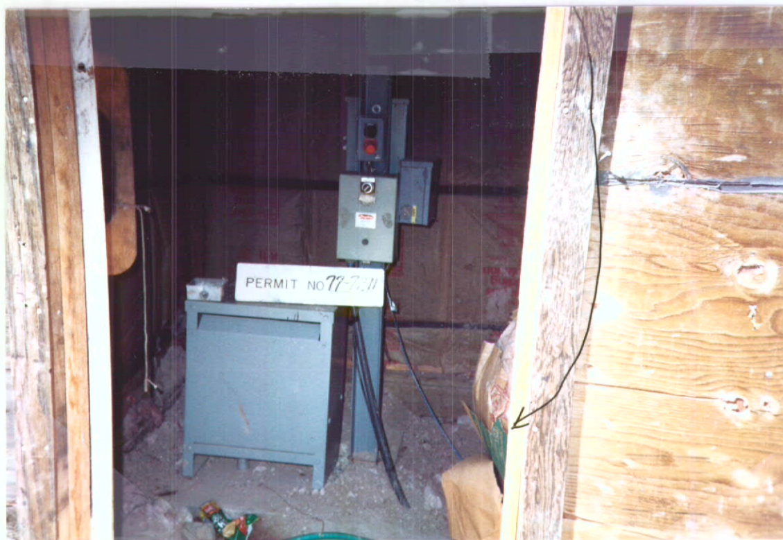
WELL CASING LOCATION
