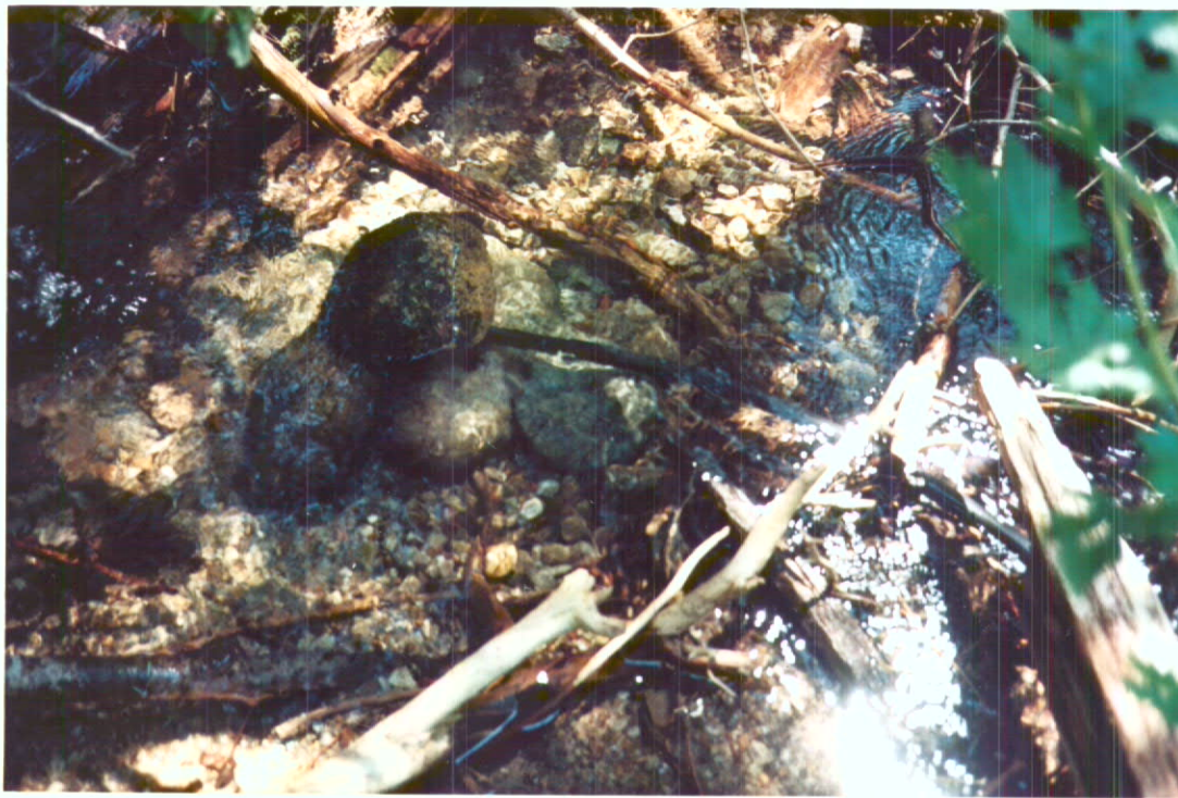
PHOTO ONE- Looking across stream, 1" black pvc line shown. Flow →
