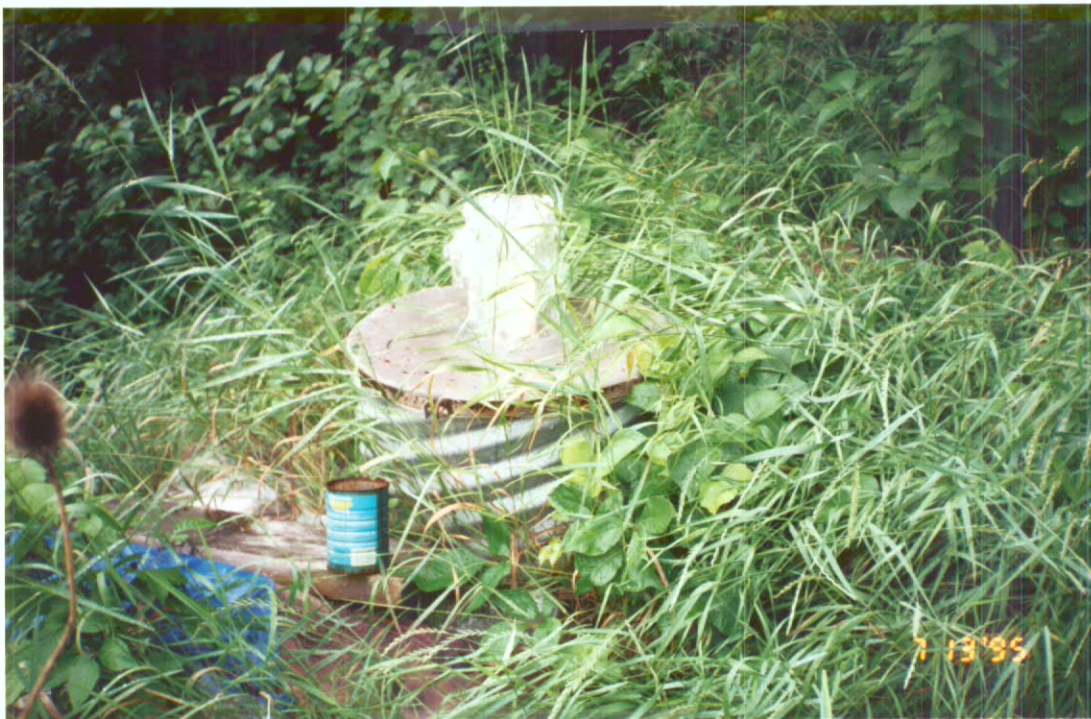
Fountain debris separator
