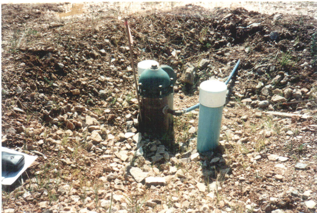
PHOTO ONE- 77-07285 well is NESENE 5.15 just east of meadow ck Landing Field.
