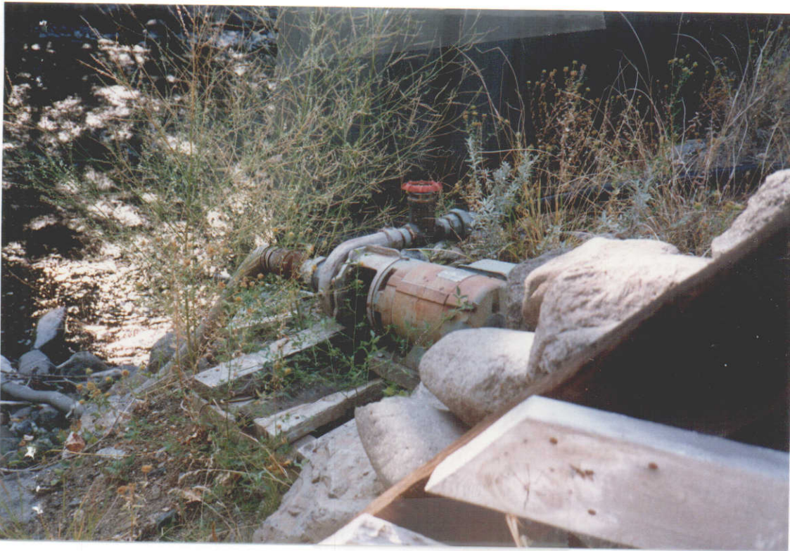
PIC. # 1 POINT OF DIVERSION FROM THE LITTLE SALMON RIVER LOOKING SOUTH WEST - NOTE BRIDGE SUPPORT
