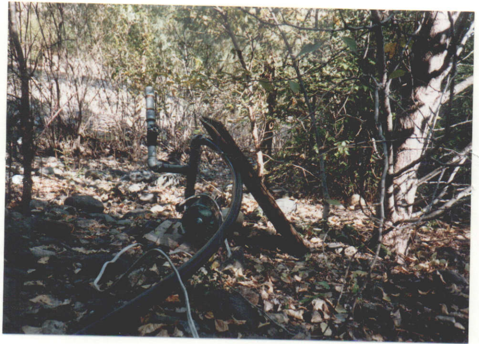
POINT OF DIVERSION NOTE LOCATION OF LITTLE SALMON RIVER THROUGH BRUSH
