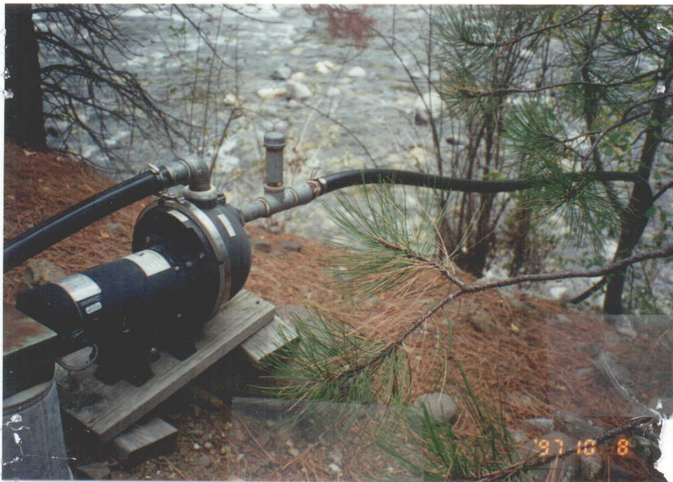
① Point of Diversion
