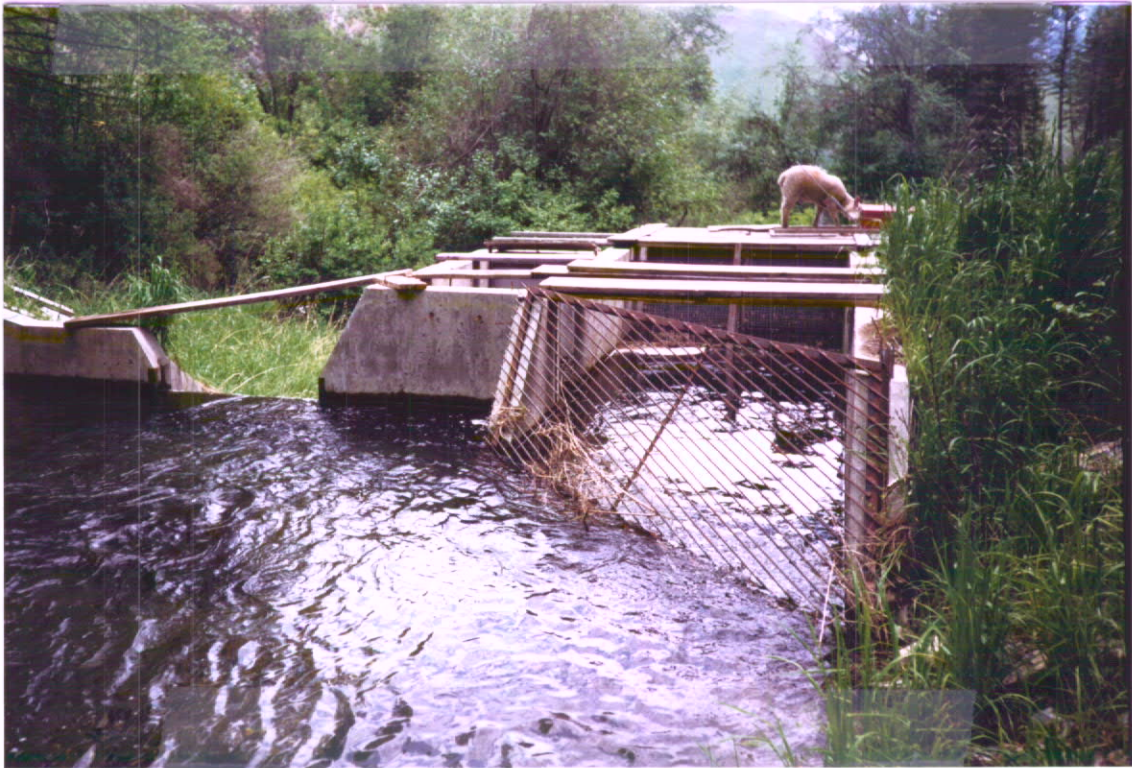
DIVERSION STRUCTURE NORTH FORK SHINGLE CREEK
