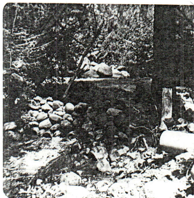
Earth Fill Dam with Penstock Diversion to Irrigation and Livestock Pond
