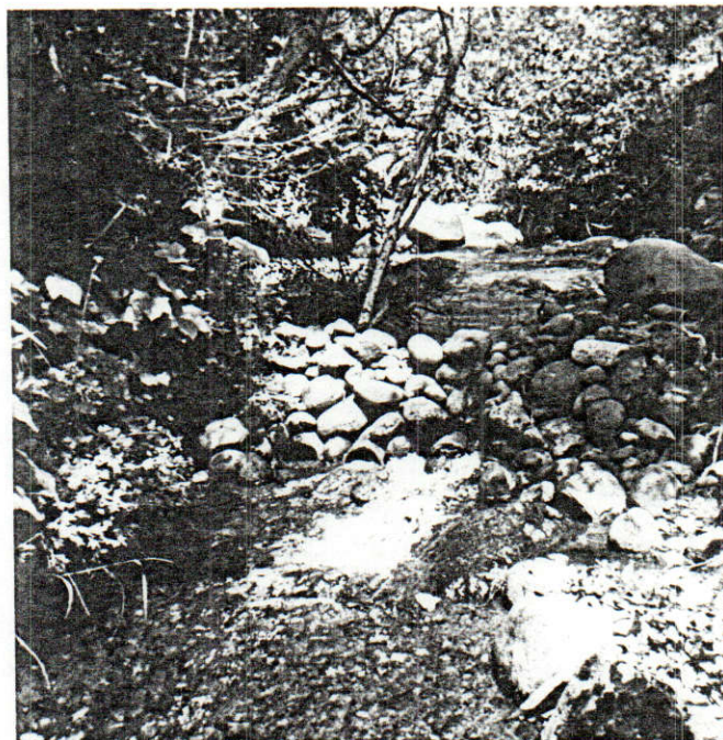
Picture of Earth Fill Dam at Point of Diversion
