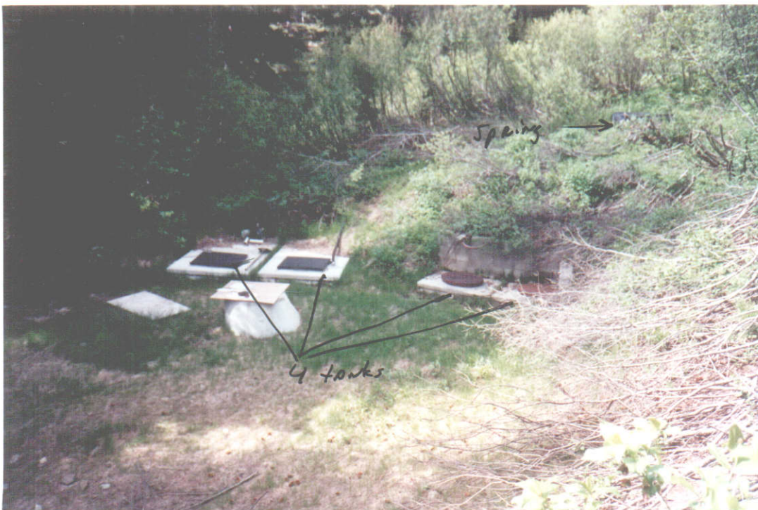
PHOTO SIX- Four storage tanks below south spring. Spring is in upper right of photo.
