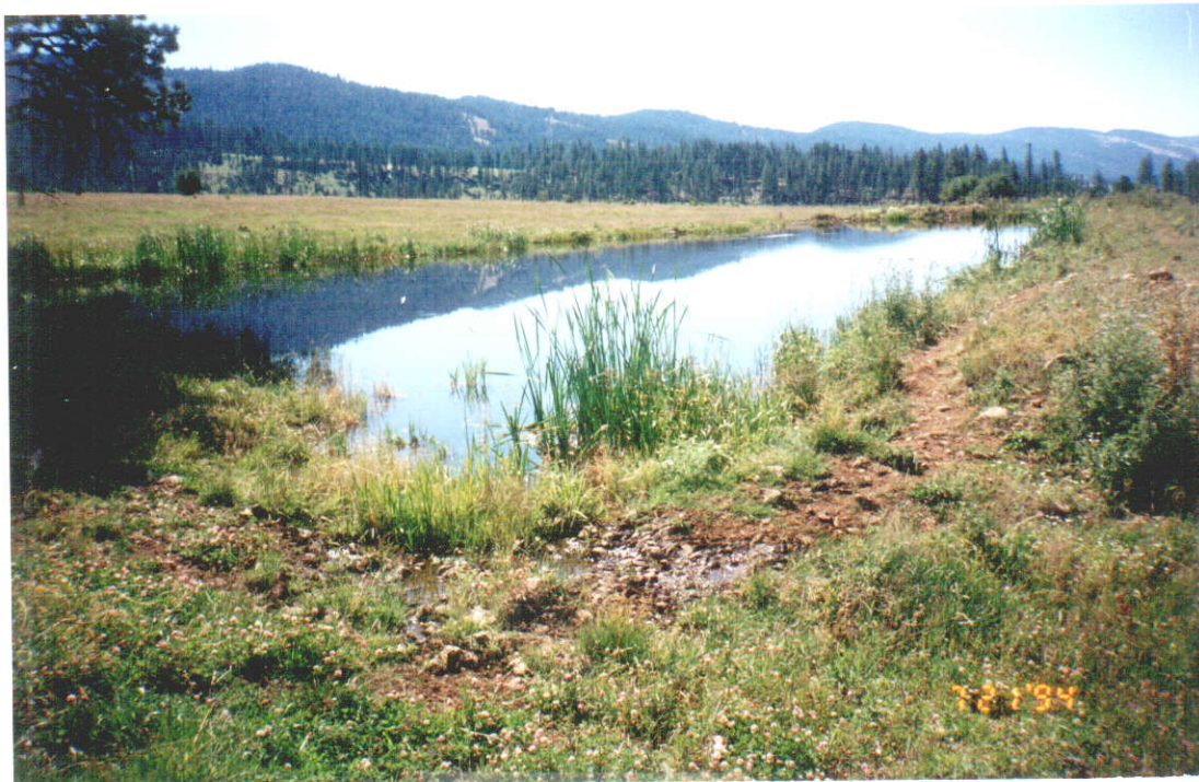
Pond #1 looking south across embankment
