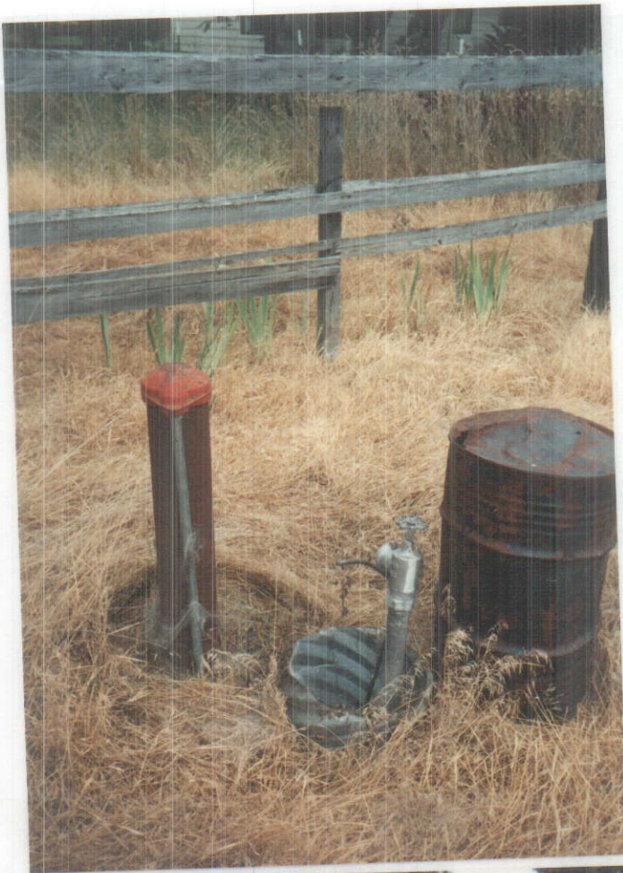
Top picture of well & pump for irrigation, riser is shown to the right of pump. Picture taken looking north east.
