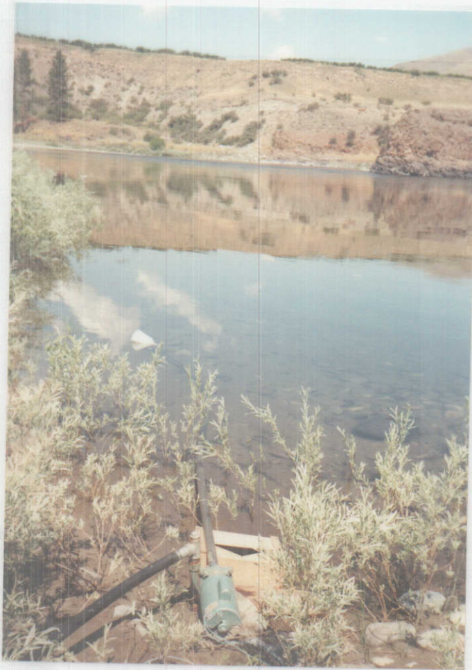
Picture of pump + main line (1.5") where water is diverted from the salmon river. Picture taken looking north.
