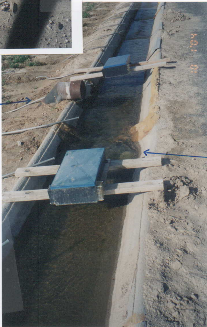
Surface water culvert entrance to property in SESW S23 TIN R2W
