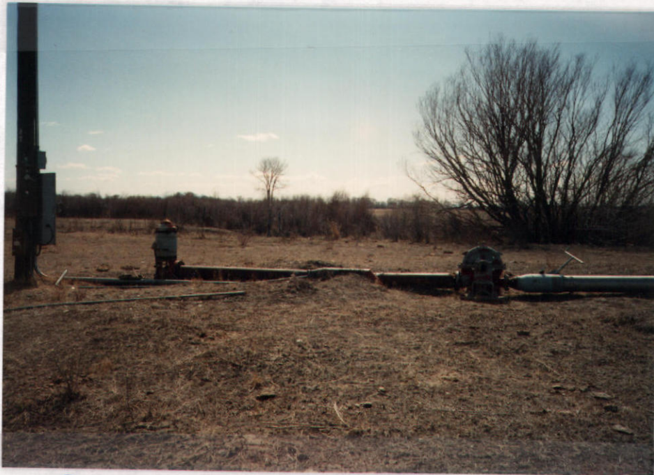
POINT OF DIVERSION "B" (VIEW 2)
