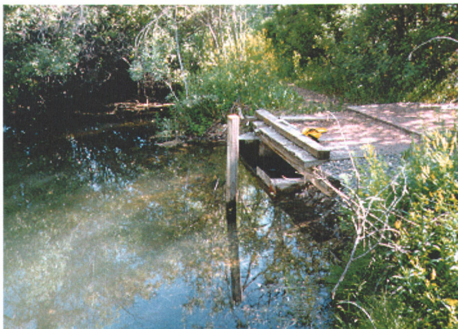
Plate 3: Weir and outlet at pond.
