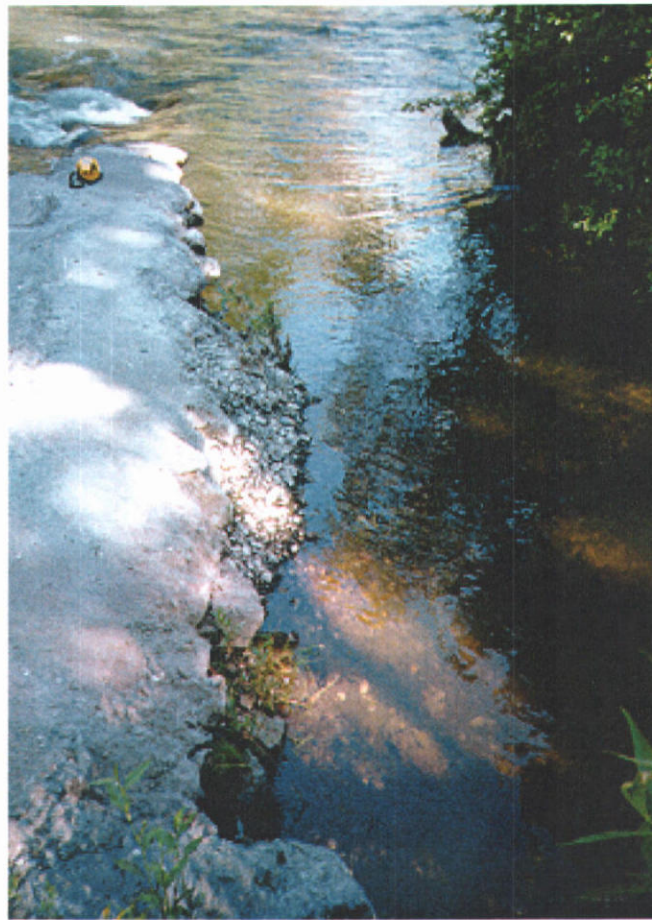
Plate 1: Diversion dam at point of diversion.
