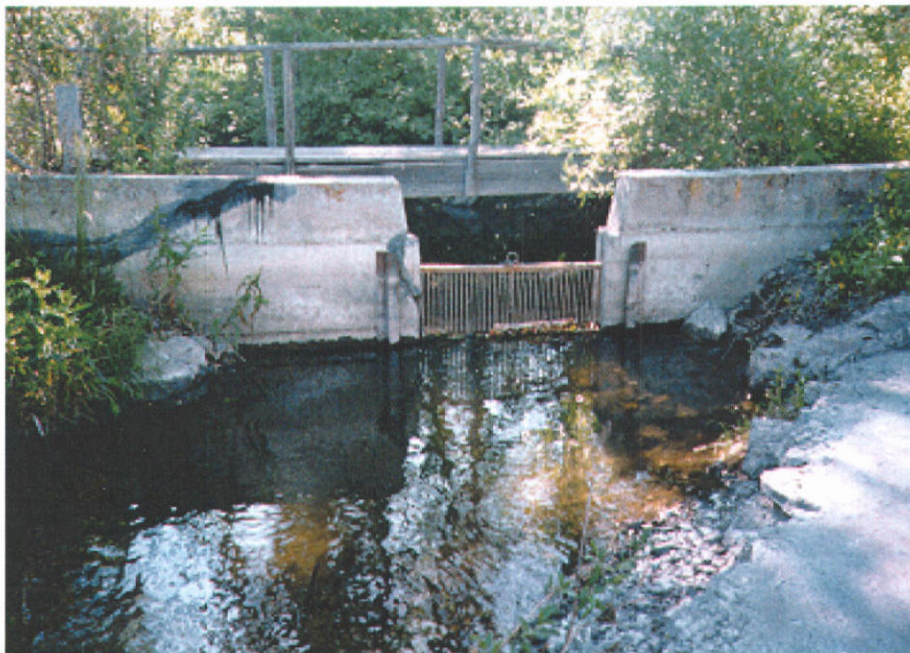
Plate 2: Headworks at point of diversion looking downstream towards pond.
