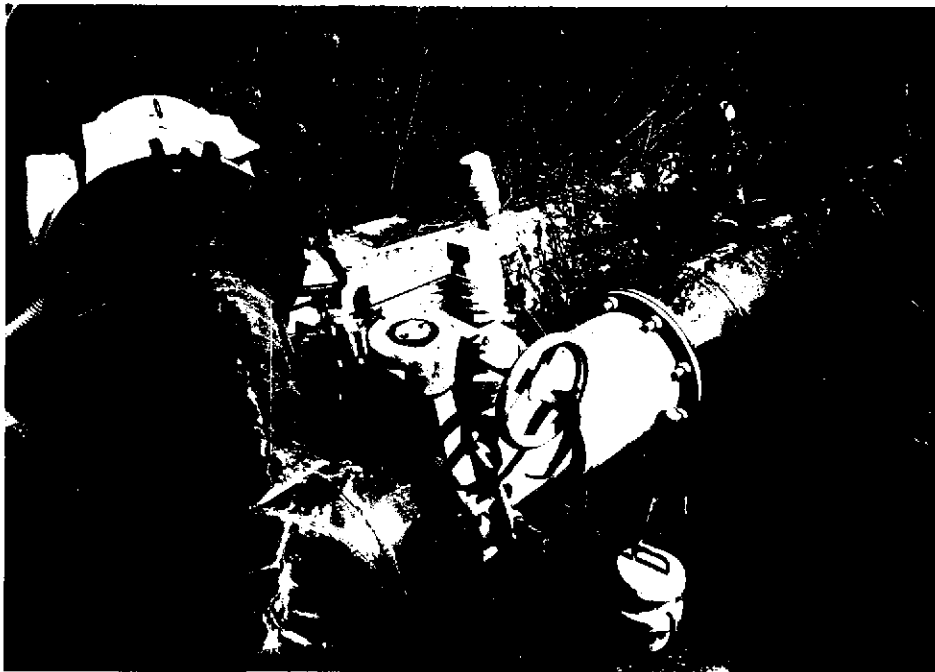
#3 West Booster Pump on Pump Station #2
