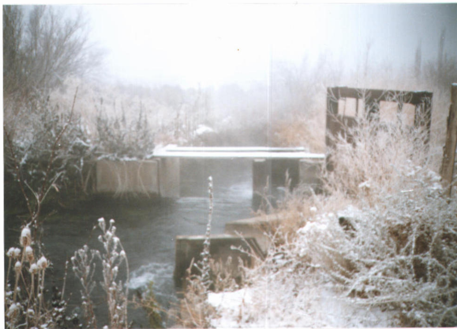
#2. Diversion works in main canal to deliver water to fish ponds.
