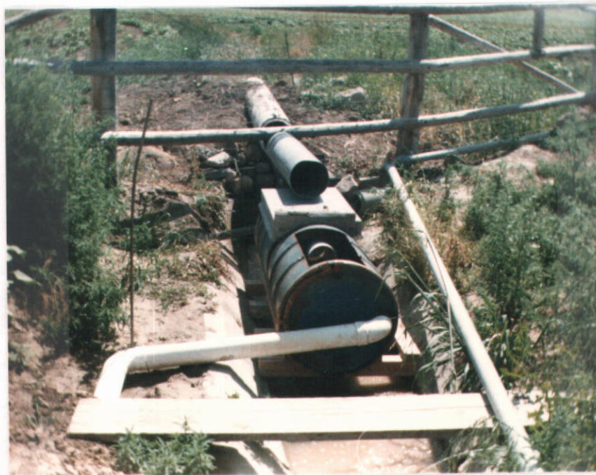
Point of diversion: A (See map) Water can be diverted into pipe on top of first barrel, through screen, barrels, and white pipe coming out of the end of second barrel, to pump A. (See below)
