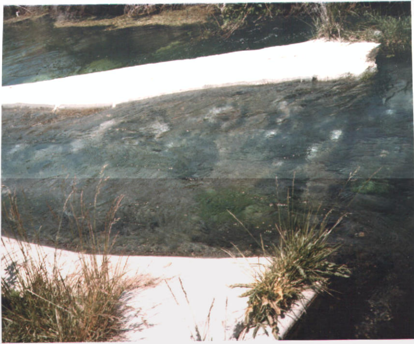
WEIR AT THE INLET OF TUCKER SPRINGS
