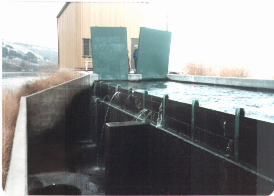
North Plant Inlet
