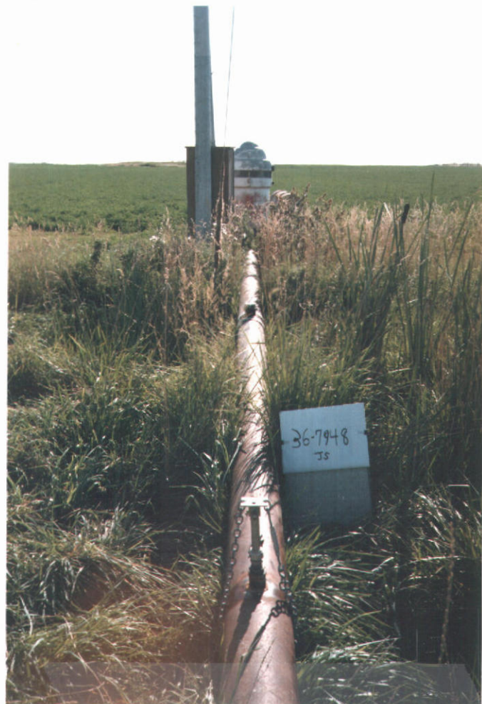
Mainline, access point
