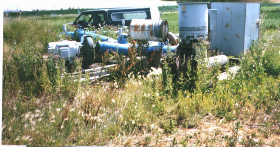
#3 Booster Pumps at Pump Station #2
