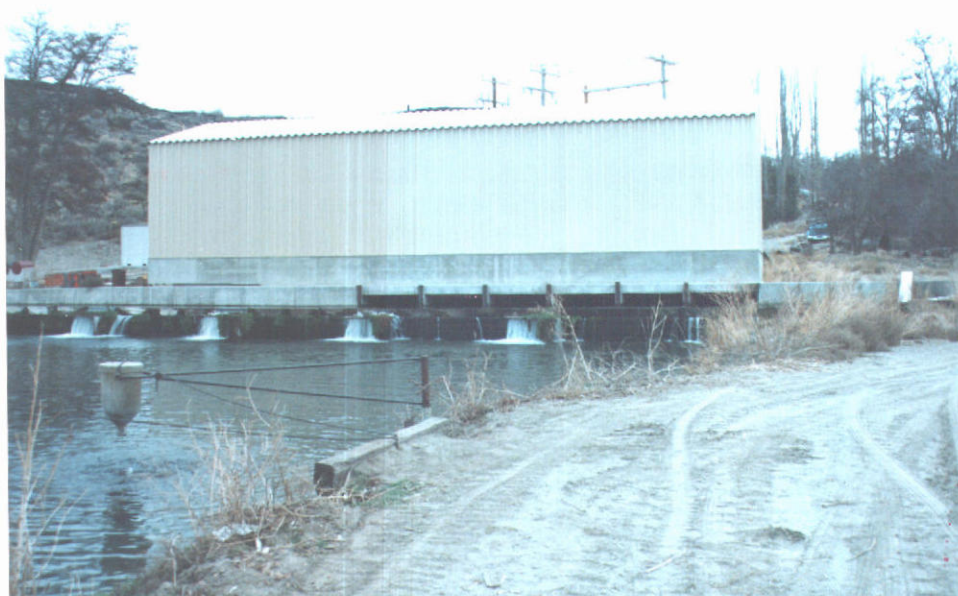
Photograph #4. Powerhouse and Tailrace Dumping into Fish Pond
