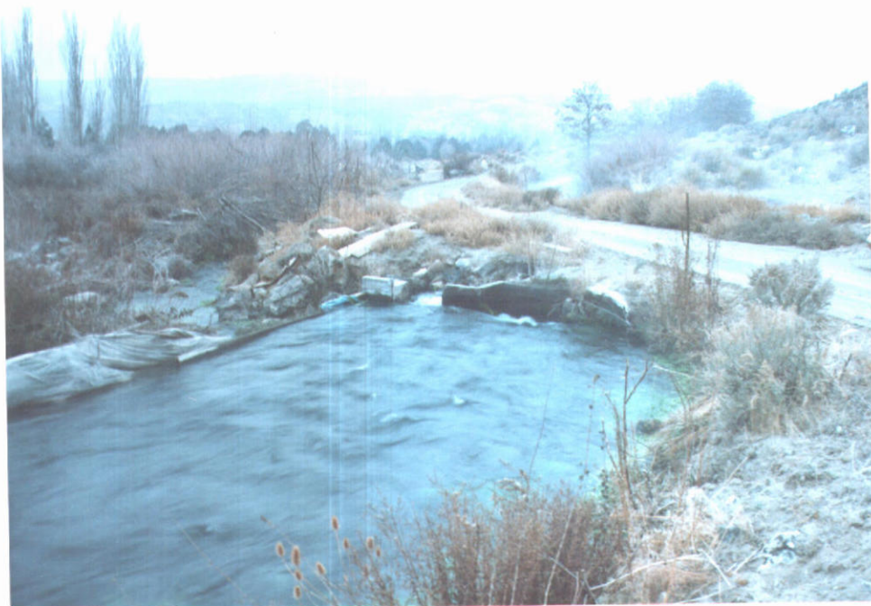
Photograph #1. Brigg's Creek Diversion to Canal
