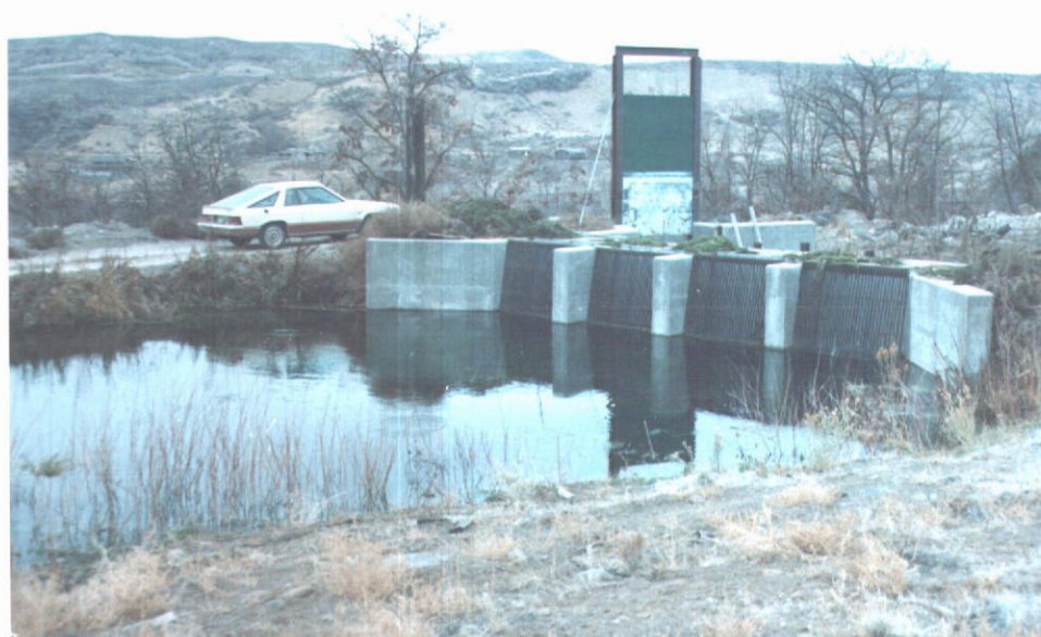
Photograph #2. Canal to Penstock Diversion Structure
