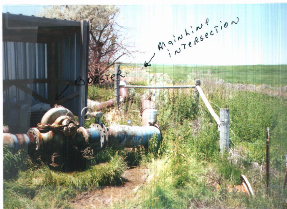
BOOSTER FOR Idaho Youth Ranch Big well. APR 15 1938 main line travels due west the joins main line leading to irrigation system
