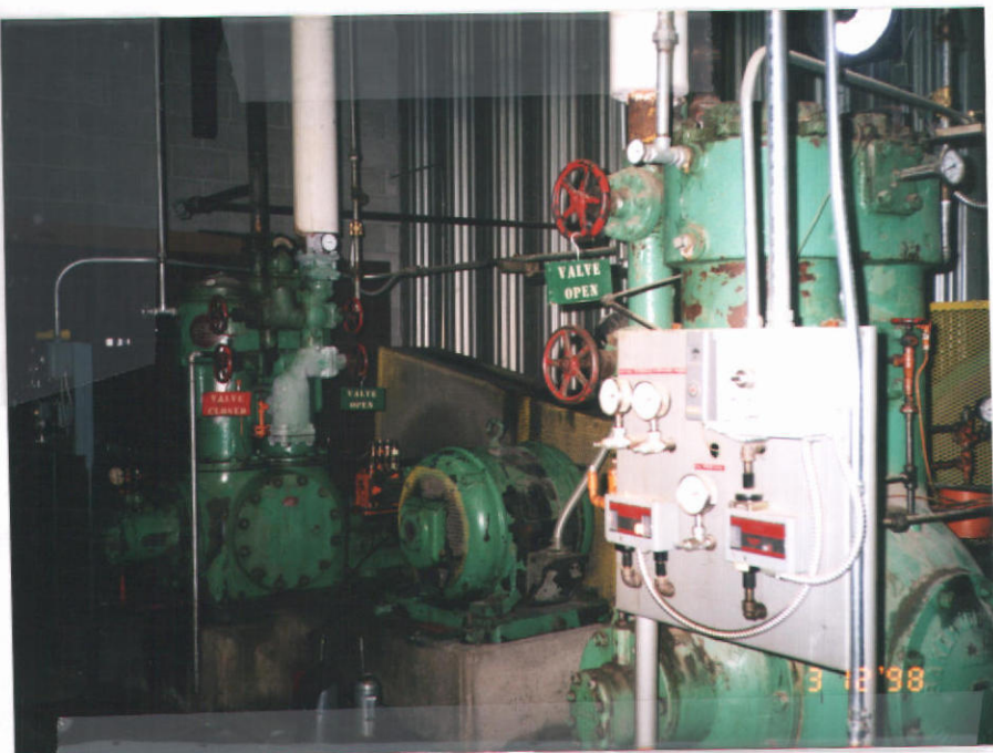
ammonia compressor, used for the cold storage
