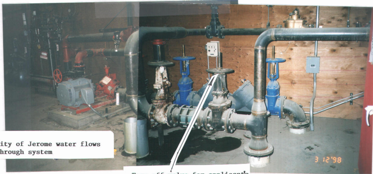
Turn off valve for applicant's p/d and city's p/d
