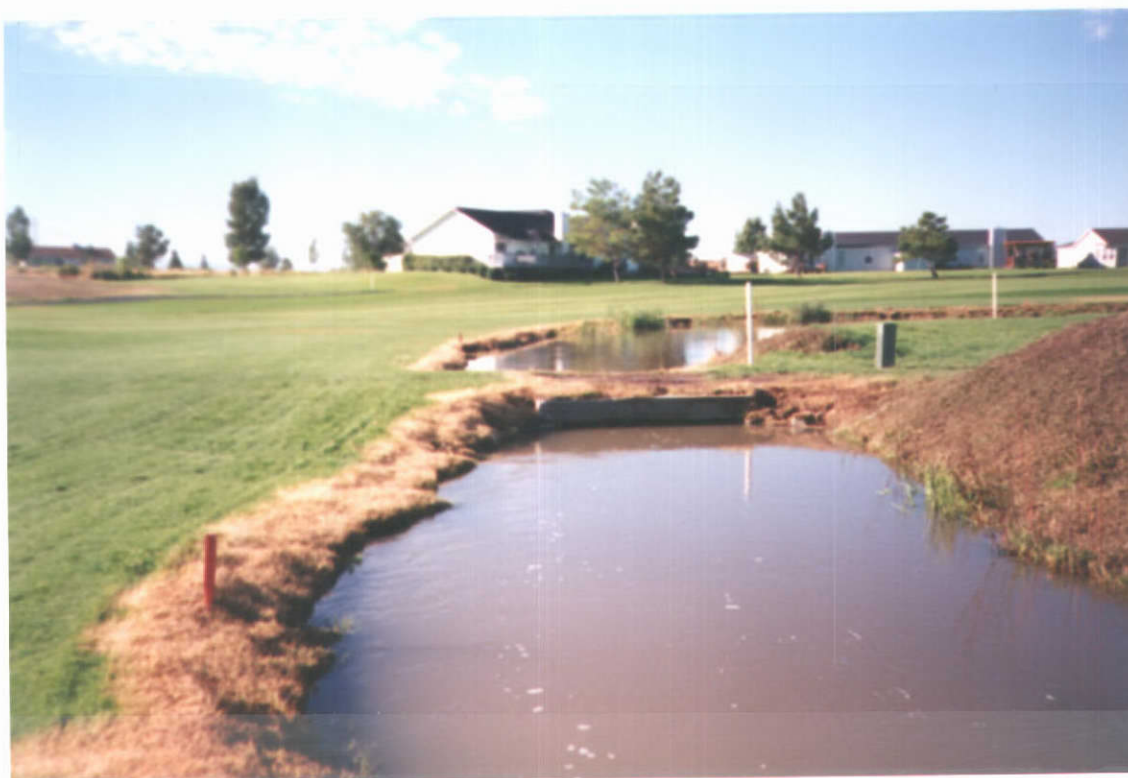
Canal Below Measuring Device
