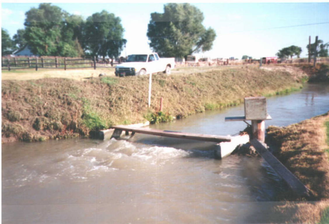
Main Canal/Waste Ditch w/Measuring Device
