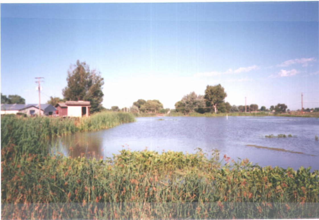
Storage Pond. Relift Pumps In Brown Building.
