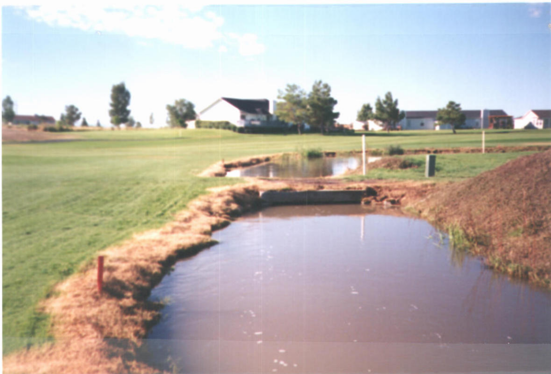
Well Discharges Into Canal Near Bridge
