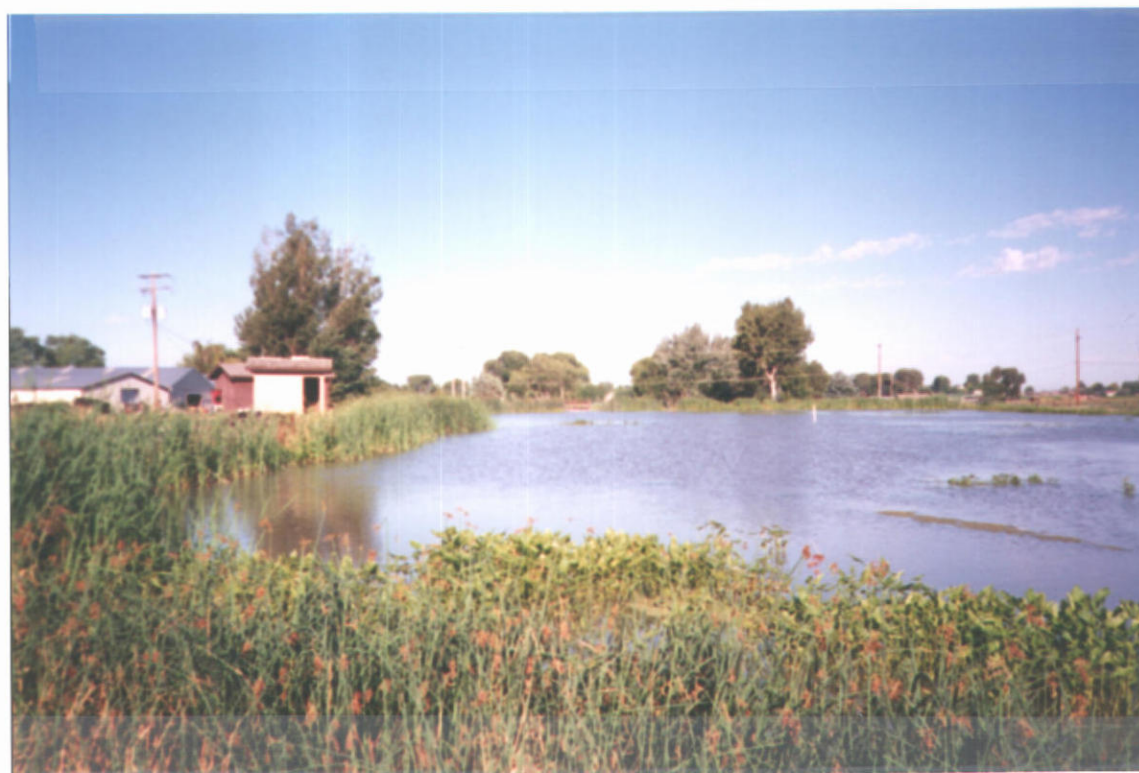
Pond, Brown Pump house (Ten Pump house for Homeowners Assn.)
