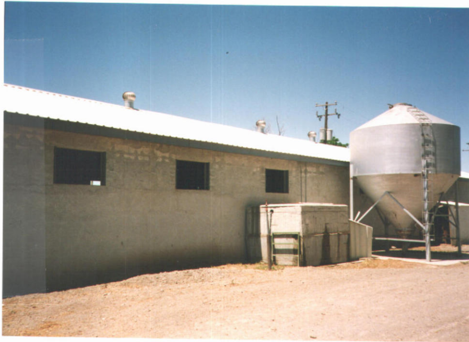
PIU - DAIRY BARN + 1500 GAL CONCRETE TANK
