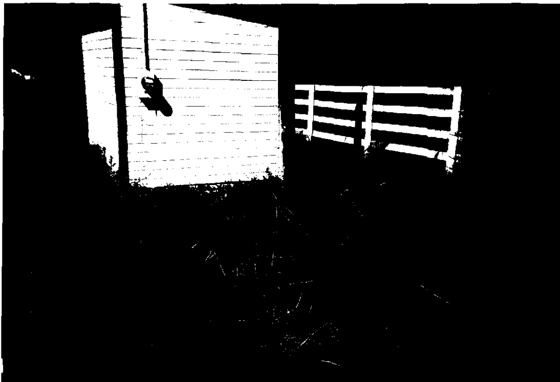
Well #3, Pump house
