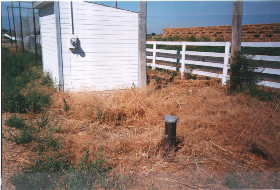
Well #3, Pump house
