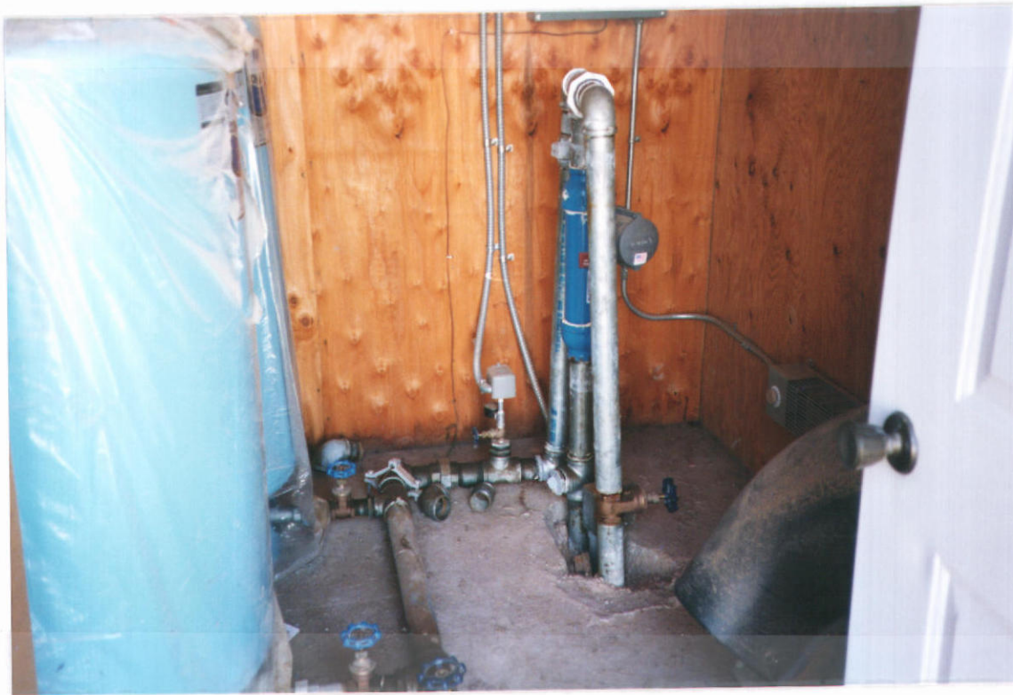
Inside Pump house
