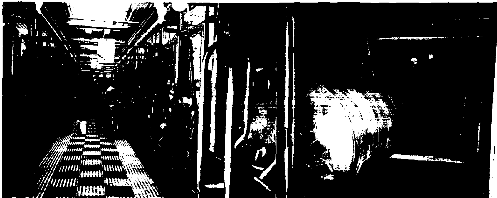
Pressure Tank w/Booster pump.
