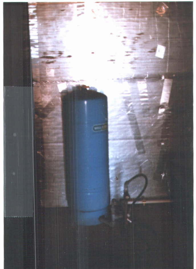
PRESSURE TANK - SOUTH #2 30 gal POTATO STORAGE BUILDING
