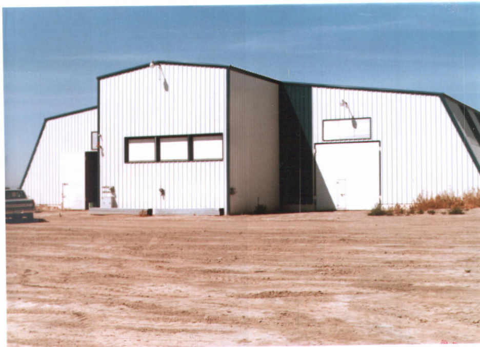
PLACE OF USE - SOUTH POTATO STORAGE BUILDING
