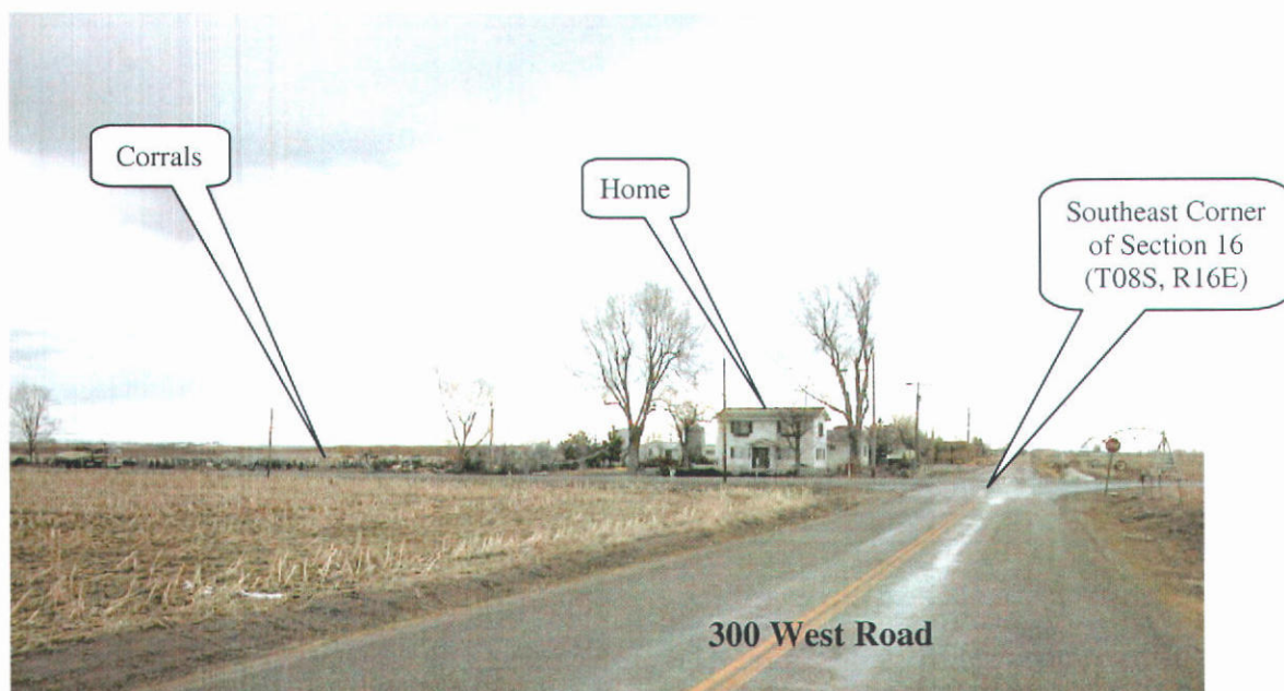
ABOVE: View looking north along the 300 West Road showing the location of the dairy site in relation to the Southeast corner of Section 16.
