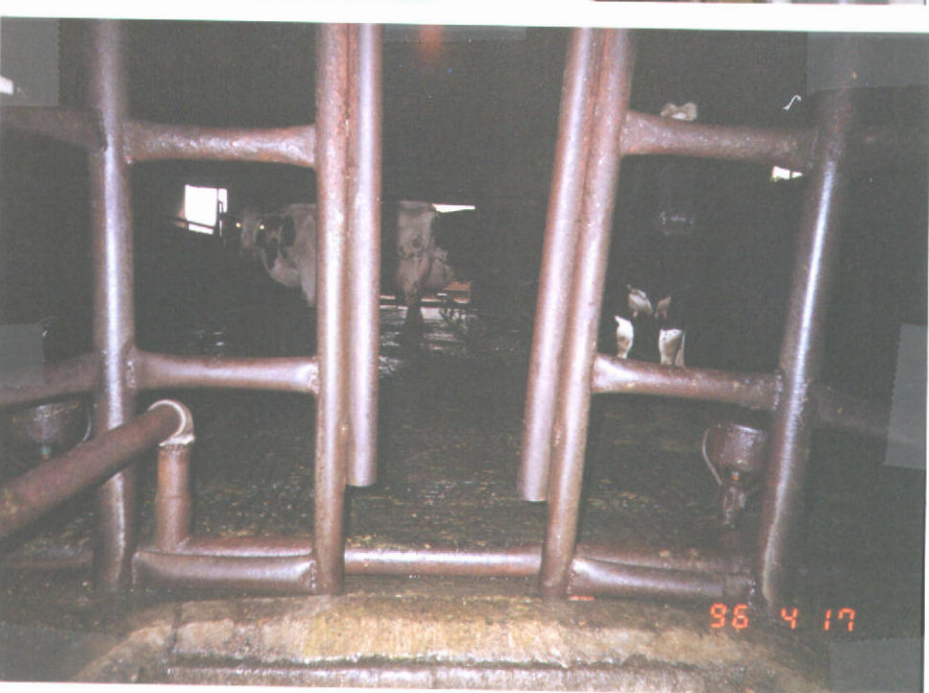
VIEW LOOKING WEST THROUGH HOLDING PEN ON WEST END OF BARN. HOLDING PEN HAS A SPRINKLER WASHING SYSTEM ON FLOOR.
