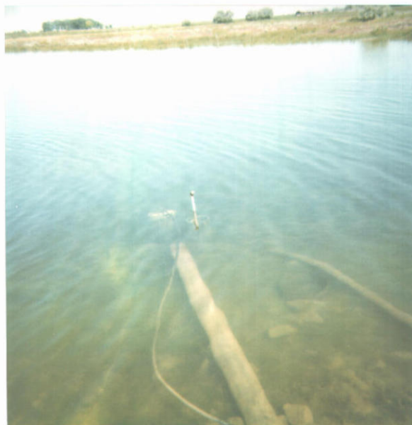
Inlet From Pond To Relift Pumps
